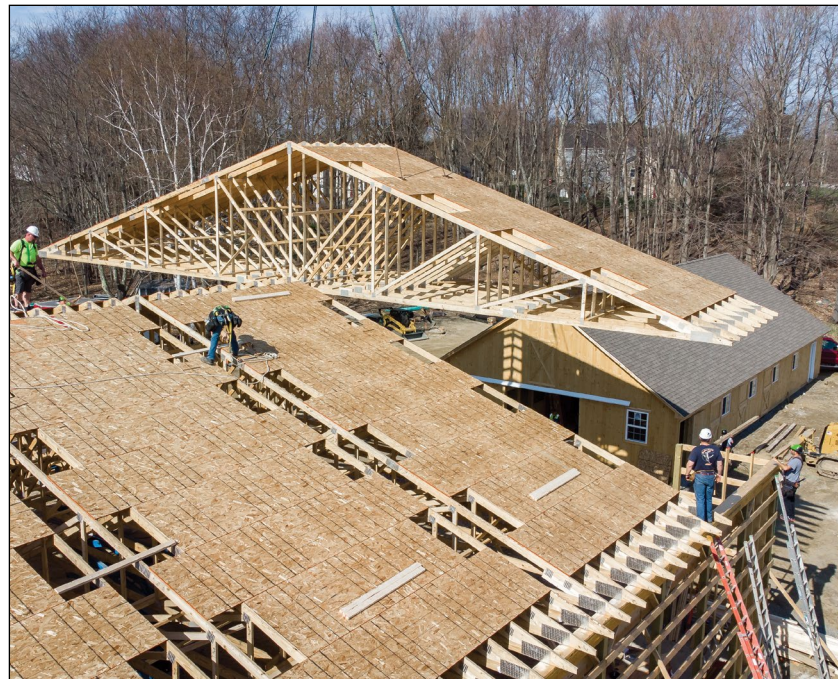
The trusses are secured on top of our new indoor riding arena.
